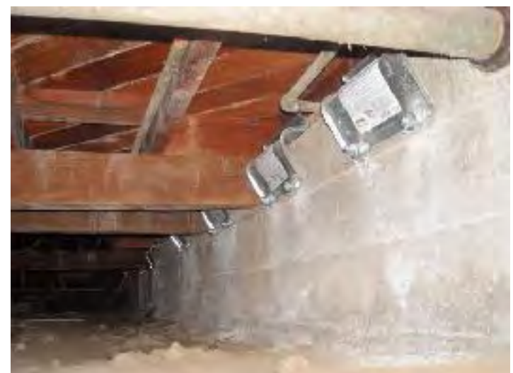
No Cripple Wall Example - UFP only
