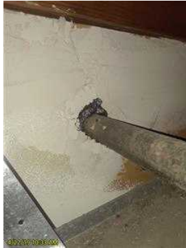
Construction gap sealed
