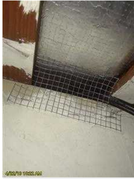
Construction gap sealed
