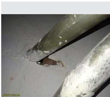
Construction gap
