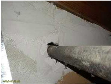
Construction gap
