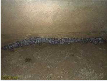
Construction gap crawlspace sealed
