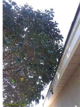
Trim away trees from roof line 3 to 5 feet
