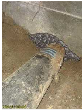
Construction gap crawlspace sealed
