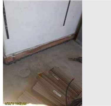
Construction gap 5 feet sealed
