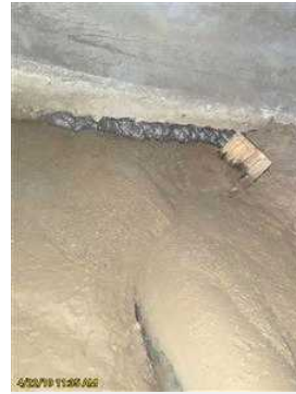
Construction gap crawlspace sealed
