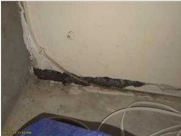
Construction gap sealed
