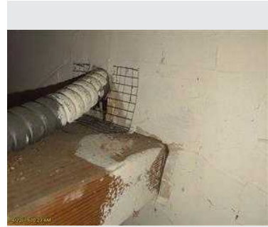
Construction gap sealed
