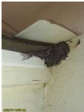
Construction gap sealed
