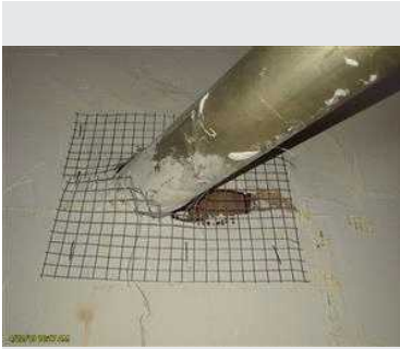
Construction gap sealed
