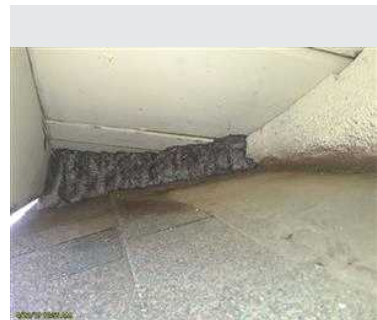
Construction gap 5 feet sealed
