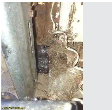
Construction gap sealed
