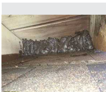
Construction gap sealed
