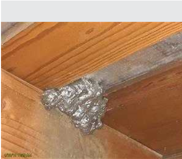
Construction gap sealed
