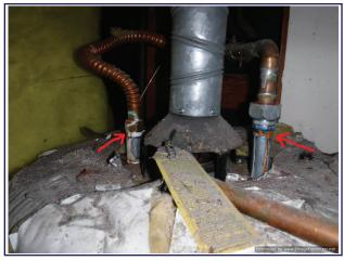
Signs of past leaking at the water heater supply lines
