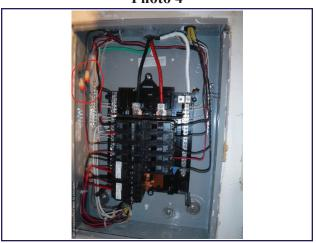
Running wire splices in the subpanel
