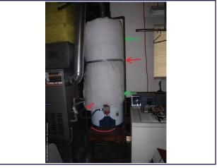
The water heater with one strap of plumber's tape for seismic restraint
