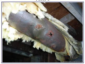
Heat duct in the sub-area with missing insulation, corrosion, and holes
