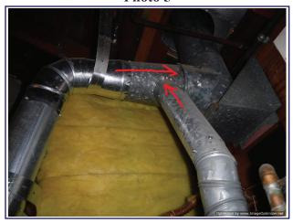
Inefficient "T" flue junction between the furnace and water heater
