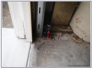
Garage door opener safety reverse sensors installed low
