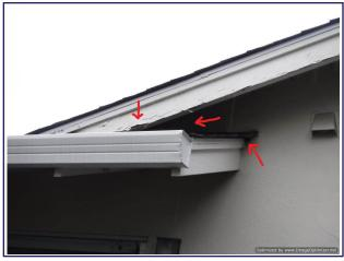
Damaged trim paint, roof edge stucco gap, and roof overlap gap
