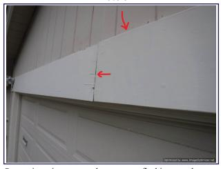
Separating trim seam and no counter flashings on the top of the trim
